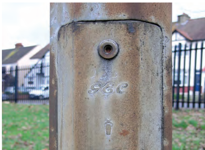
Close-up of the microphone symbol on an access plate near the bottom of the mast
